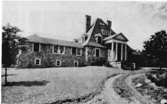
"Dogwoods," the Main House on the Homestead. One of the Wings Contains the Workshop, the Other, the Loom Room. Designed and Built by Amateur Labor. Even the Wiring, Plumbing, and Steamfitting Were Done by What Can at Best be Described as Semi-skilled Labor. The Stonework in All the Houses on "Dogwoods" Was Put in by Amateurs, Using a Modification of the Flagg Method of Wall-building.
